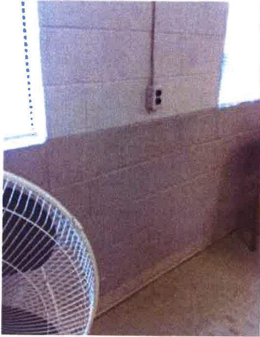
BASEBOARD TO BE REPLACED
