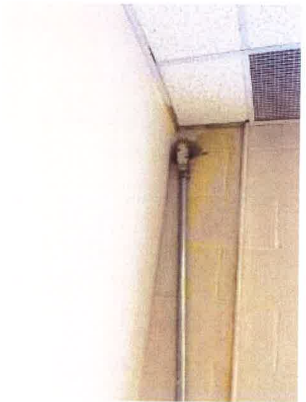
HOLE IN EXTERIOR WALL
