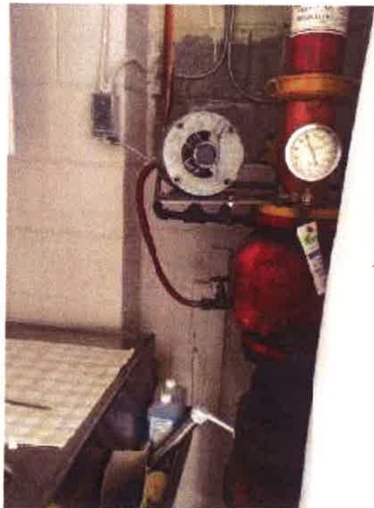
SPRINKLERS MANIFOLD TO BE ENCLOSED
