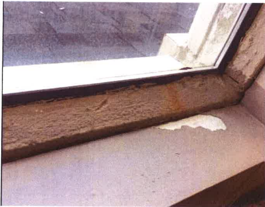
'THERMAL BRIDGE' BETWEEN INTERIOR AND EXTSRIOR MAKES INSULATION INEFFECTIVE
