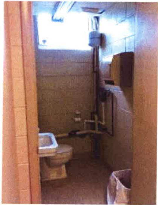
PIPING TO BE ENCLOSED INTO WALL SPACE
