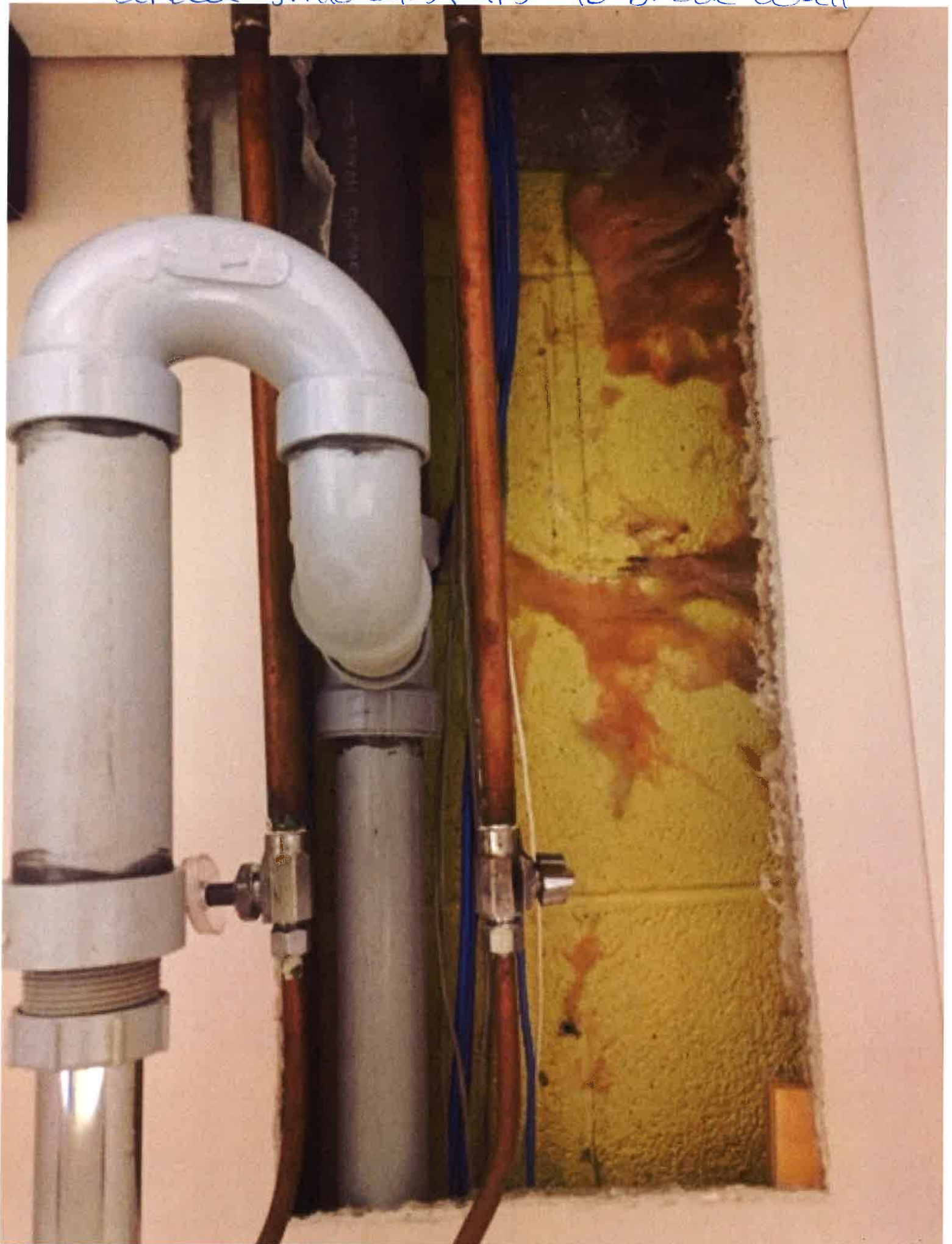
Under Sink upstairs to Block Wall
