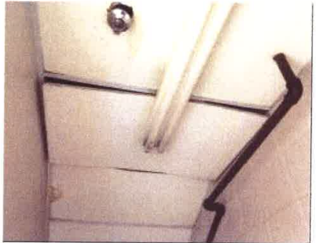
CEILING IN STAIRCASE
