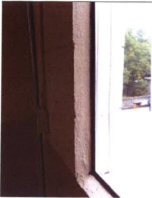
NO THERMAL INSULATION IN EXT. WALLS
