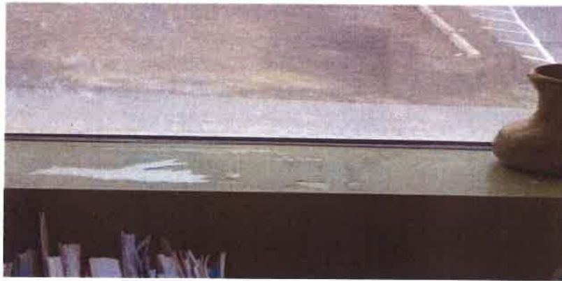
RESULTS OF CONDENSATION ON WINDOWS
