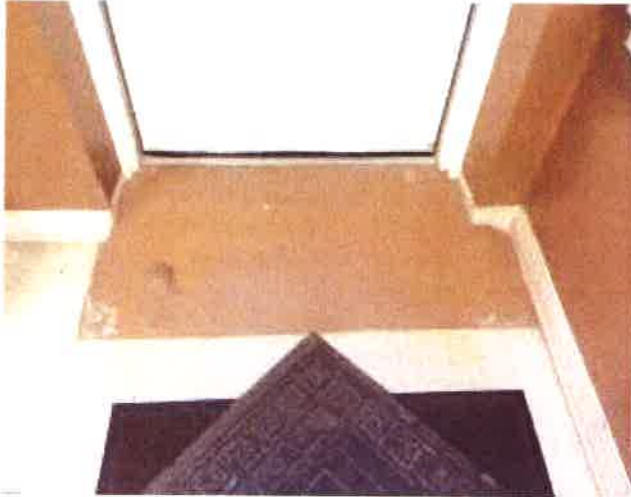
BARRIER- FREE RAMP AT DOOR
