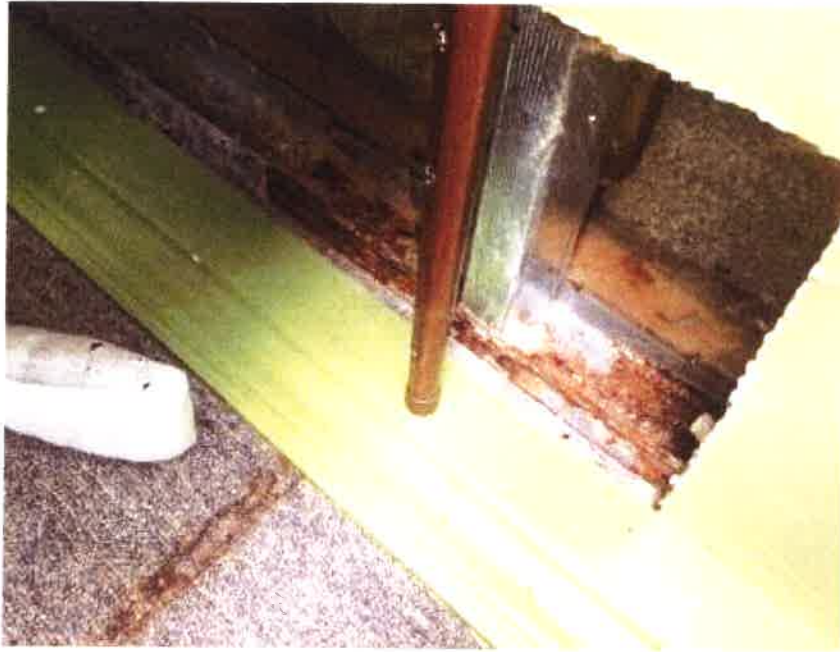
WATER DAMAGE IN WALL
