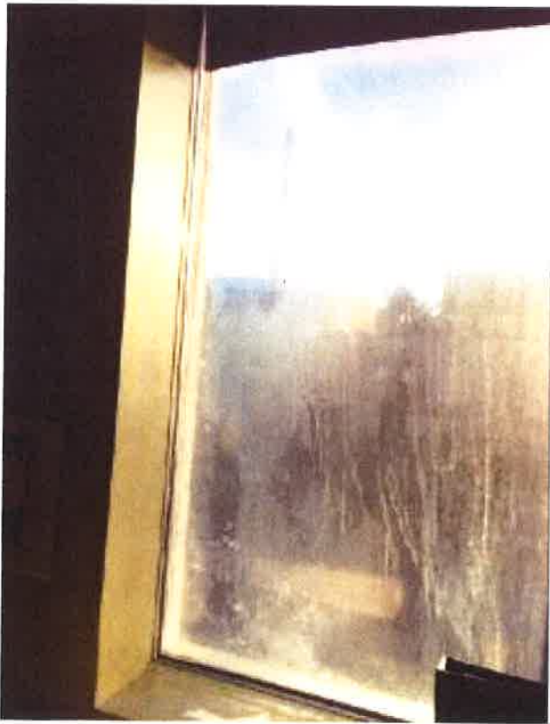
BROCKEN THERMAL SEAL ON WINDOW
